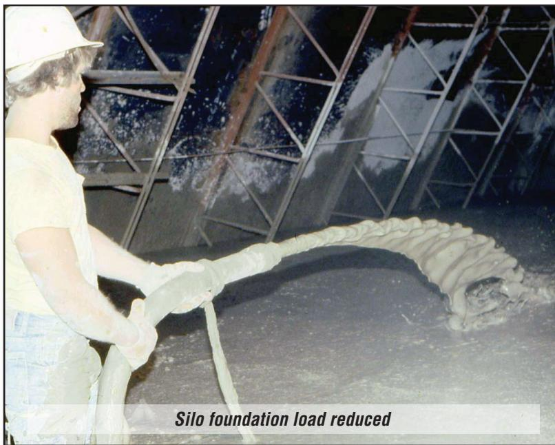
*Elastizell EF fills the voids (seen in orange at right) behind the sloping discharge hopper plates and the slipformed silo wall.*
